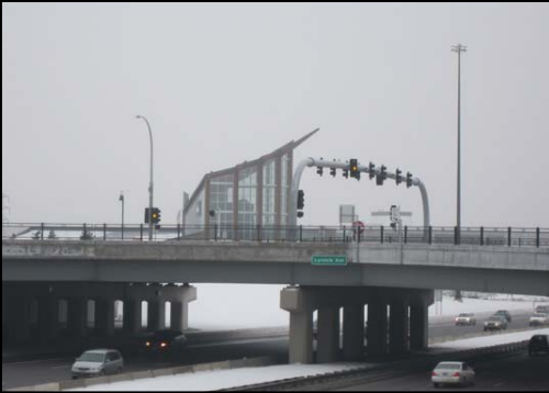
The new Lyndale Avenue bridge features a single point urban diamond configuration.
