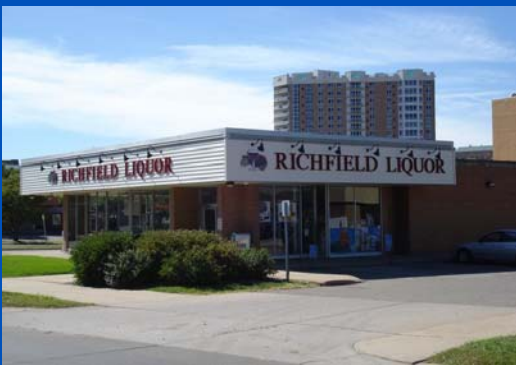
Lyndale Liquor Store received an upgrade in its signage.
