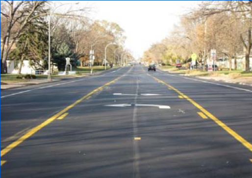
Portland Avenue was converted to 3 lanes between 68th Street and 78th Street.
